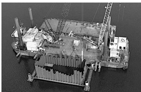
Figure 1. Steel caisson in foreground and barge with pile driving and compaction equipment in background.
